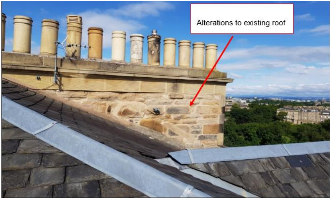
Figure 3: previous alterations to the original roof of no. 10 Randolph Crescent facing rear (north), as evidenced on chimney stack.
